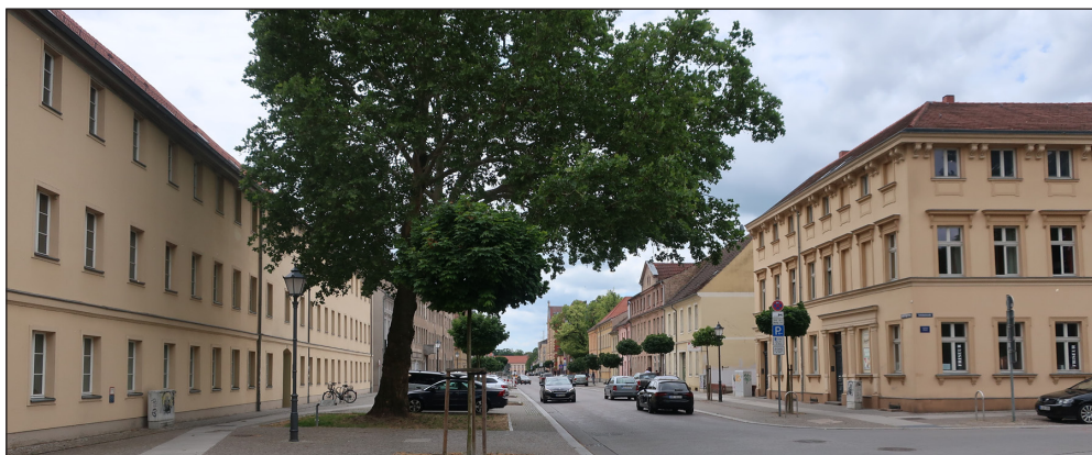
Figure 2: Neuruppin in 2019 still exhibited the principles guiding its rebuilding after 1787: wide streets, open spaces, tile roofs, evenly spaced windows, and the absence of wood. Photographed by the author.
